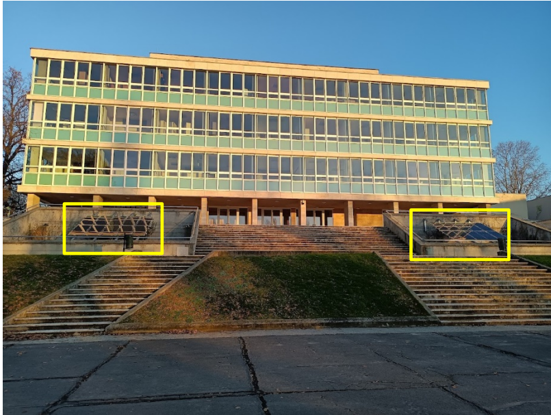
Figure 4. The location of the semi-transparent photovoltaic PV system
