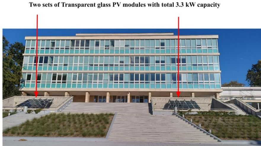
Fig. 3.4. A 3.3 kW transparent glass PV module at the entrance of the Aula building
