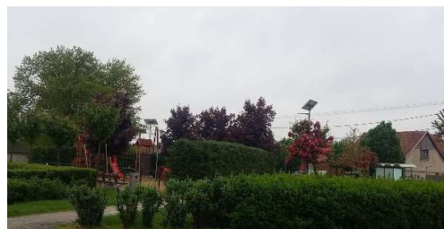
Figure 34. Solar panels on lamp post, Gyál, Hungary.
