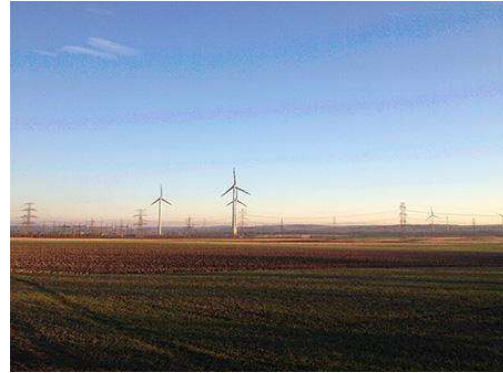
Figure 42. Wind turbines in Burgenland, Austria.
