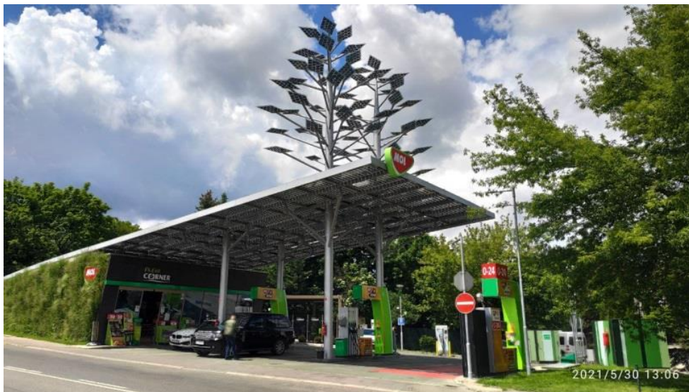
Fig. 2.4. MBSS used for powering fuel station (Budapest, Hungary)
