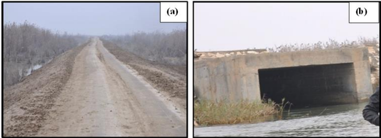
Figure 7: The security dike through Al-Hammar marsh, Aug. 2019 (a) General view, (b) One of the culverts under the dike.
