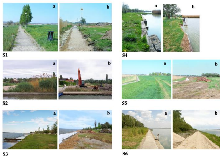
Figure 4.8 Comparative photos of the lakeshore before and during construction
