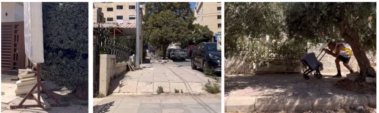
Figure E14. blocked path throughout site D showcasing blockage of trees and unfixed paves.
