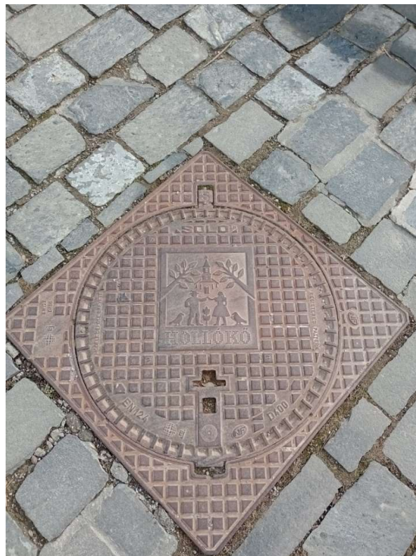
Figure 65. Hollókő's Manhole and Underground System Source: Author, 2023
